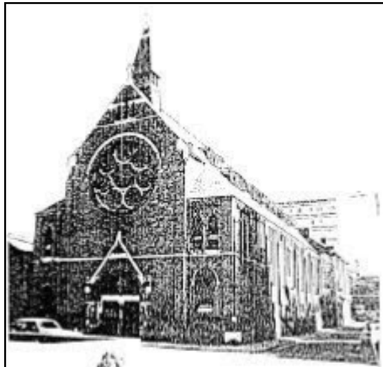
St Alphege, Southwark, demolished in 1991.
