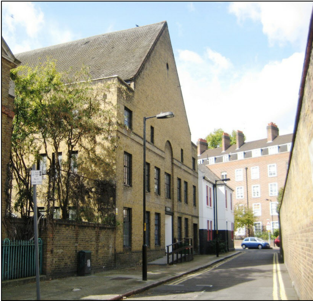
St Alphege's entrance on King's Bench Street. The Oratory of St Alphege is at the junction with Pocock Street (painted white and black).
